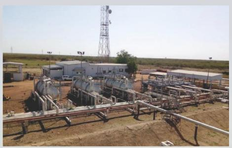
Free Water Knock Out Drums and plate heat exchangers at FPF
